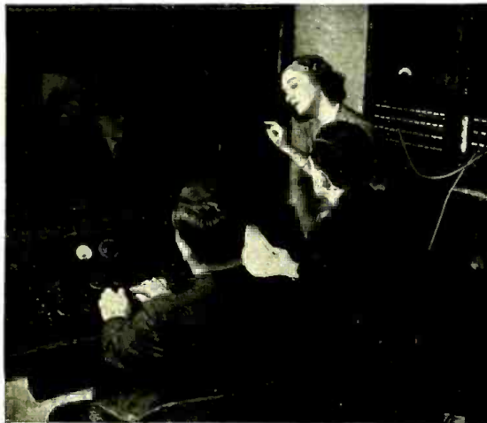
2 —CONTROL ROOM—Miss Blackburn, however, doesn't stick around for that. Instead she goes to the control room and watches the engineer manipulate the "mixing panel" by which the proper volume and intensity of sound are blended.
