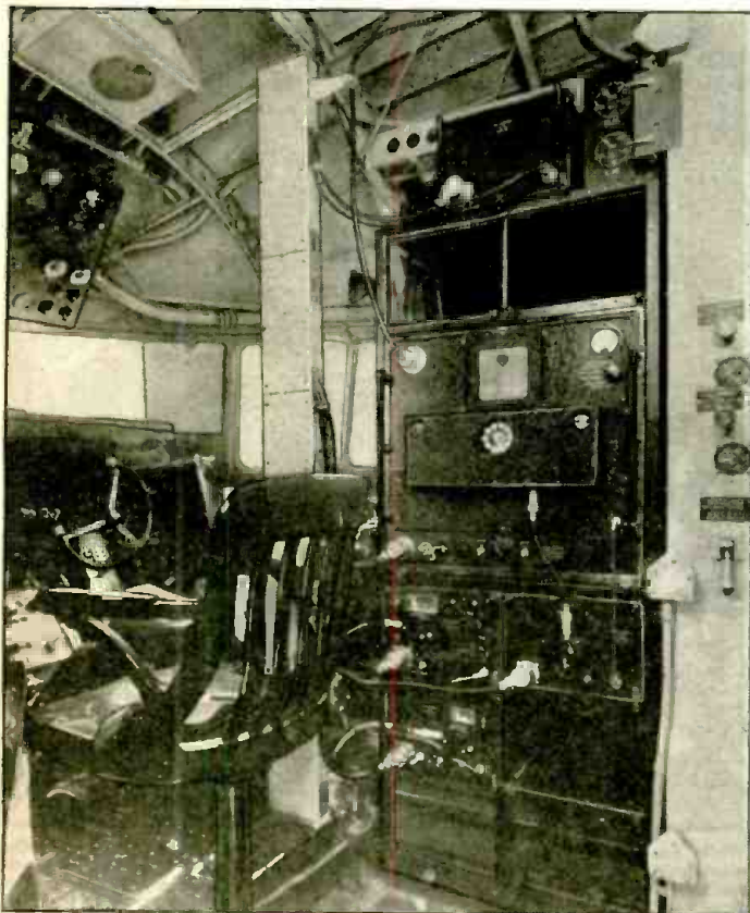
Eleven units of radio equipment will ultimately guide the giant DC-4; only 5 are shown here. The radio rack holds (top) the inter-communicating system amplifier; (next lower) the 250-watt transmitter joined through flexible shafting to the communications receiver below it. The auxiliary receiver is seen immediately to the left of the latter unit and below it is the beacon receiver. When aloft, radio operation is governed remotely by a control column.
