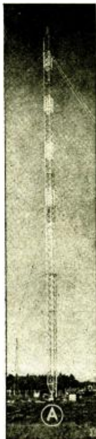
A HALF-MILLION POUNDS OF STEEL RISES HIGHER THAN WASHINGTON MONUMENT. Completion of WGY's (Schenectady, N. Y.) new 625-foot vertical antenna, last month, gave General Electric's 50,000-watt "voice" sufficient strength to effect a 40% increase in service area. The spire, painted in alternate stripes of orange and white, is topped by a 1,000-watt flasher aviation beacon; constantly glowing lights (automatically turned-on by means of photo-electric cells upon the approach of darkness!) are spotted at different levels. The completed tower (A) passed through important transitional stages. For instance, in order to test the ground upon which the concrete mounting block was to be placed, pigiron was piled onto the spot until a pressure of 8,000 lbs./sq.ft. was exerted, and ground-settling measurements made for a month; yet, the actual tower exerts a pressure of only 3,000 lbs./sq.ft. In order to insulate the "live" tower from this concrete block a hollow porcelain shell is used (as shown in B). A U.S. Bureau of Standards hydraulic testing machine was used to determine the strength of this shell; at about 2 million lbs. pressure (4 times normal) a duplicate test-shell exploded with a cannon-like crack (C and D).
