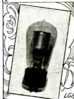
Helium Rectifier; 250 ma. Output for "A" Eliminators. About 1925-'6. LGP
