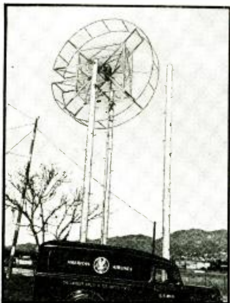
The 20 ft. loop to aid plane dispatching.
