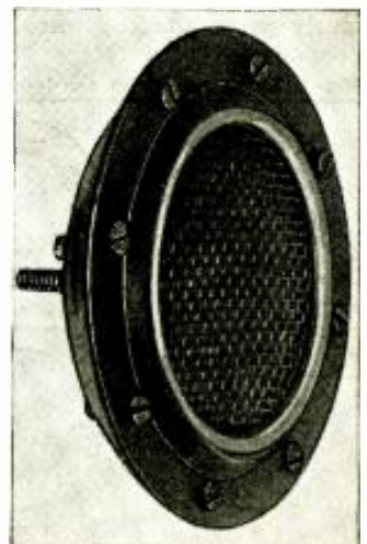
Fig. A, right. The re-made microphone closely resembles the carbon unit from which it was made. The rivets have been replaced by 6-32 machine screws according to instructions, in re-assembling it.
