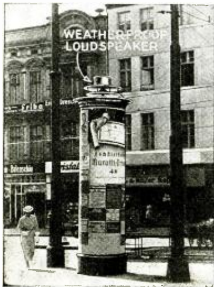
Fig. 2, above. A record grooving guide. Fig. A, below. The sign pillars in Berlin have been given a voice—via P.A.
