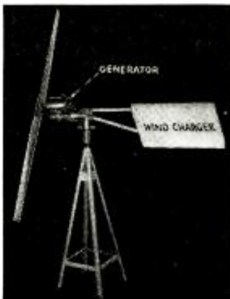
Wind-driven battery charger. (896)
