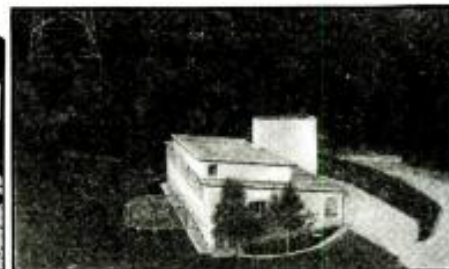
The Monte Ceneri 15 kw. broadcaster located in a remote part of the Swiss Alps.
