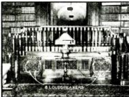
One of the many loudspeaker installations.
