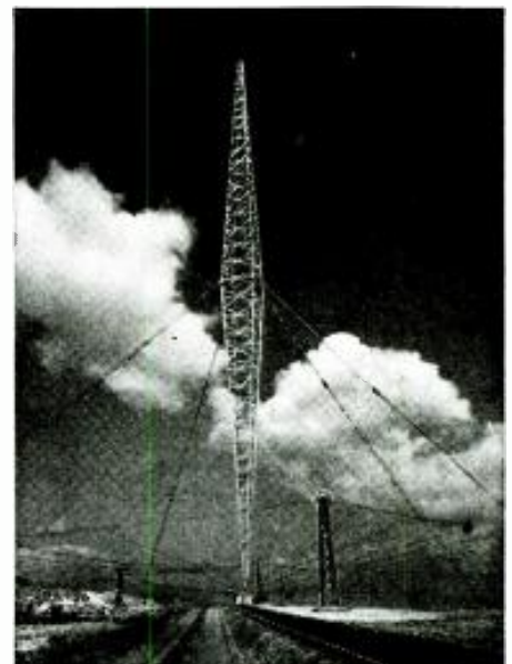
The photo at the left shows part of the aerial and the transmitter building of the broadcast station at Helsinki, Finland. Right, the aerial and counterpoise system for the broadcast transmitter at Bisamberg, near Vienna, Austria. The tower is 400 ft. high.
