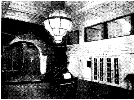
Studio of the 120kw. station at Warsaw, Poland.
