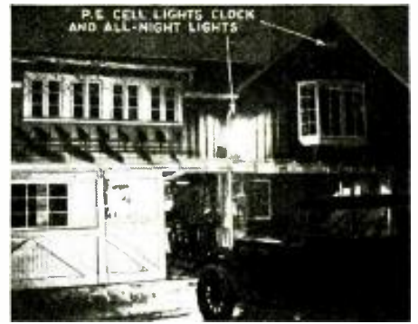
(Photos, except Fig. C, McGraw-Hill.) Fig. A, PE. cell switches lights.
