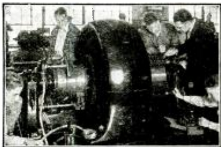
Working on Real Electrical Equipment at Coyne
