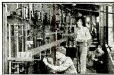
A Real Switchboard In the Coyne Shops
