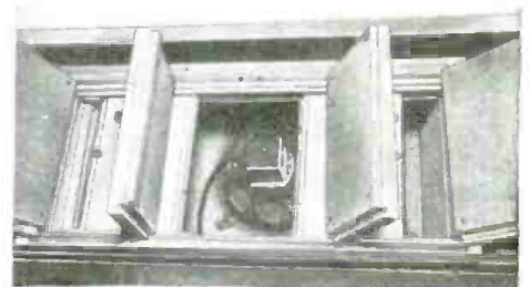
Fig. G A two-room speaker installation. When the doors on either side are closed nothing can be heard.
