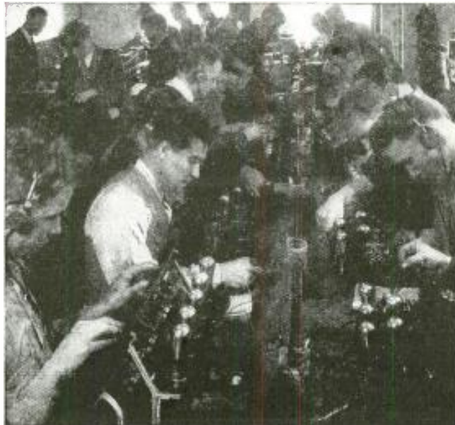
A scene in the big, busy Radio Shops at Coyne. Here you see fellows working on real Radios—not reading about them from books or lessons. This is THE way to prepare for the big-money field of Radio!
