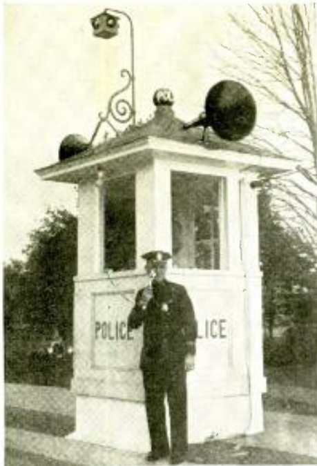
An unusual use for P.A. Amplifiers for controlling automobile traffic. This booth is used by Chief of Police William Nichols, of Stratford, Conn. Here is a great idea for Service Men to take up with police chiefs in their own towns.
