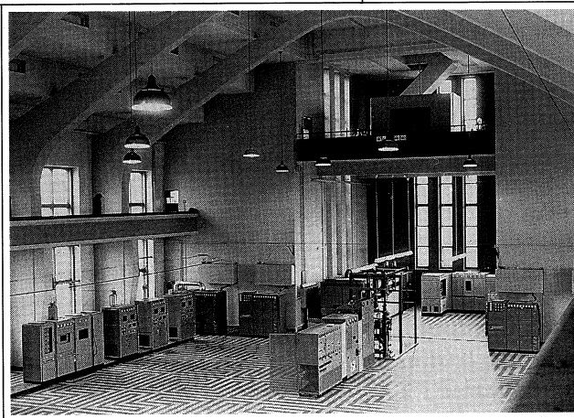
Visible at the extreme left is one of the two alternators, in the center the control desk. Behind the desk are the saturated core transformer frequency multipliers and aerial inductances. The frequency of the alternator had been changed from 6,000 Hz to 5,600 Hz, and most of the traffic was concentrated on 16,800 kHz. Consequently, some of the frequency-multiplier equipment had been removed as no longer being necessary.
