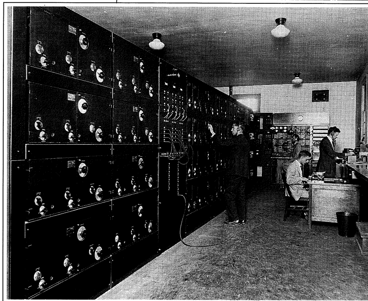
◀ Photo 9. Long wave receivers at Belfast, Maine similar to L/W receivers used at Riverhead Building #2.
