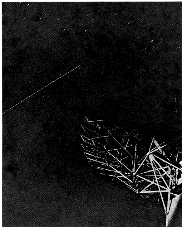
Echo I satellite, visible to naked eye as bright, fast-moving star, streaks across heavens over Bell Telephone Laboratories' "dish" antenna at Holmdel, N. J. The 60-foot antenna was used in the first space communication experiments during 1960.
