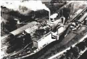
Lehigh Portland Cement, Allentown
