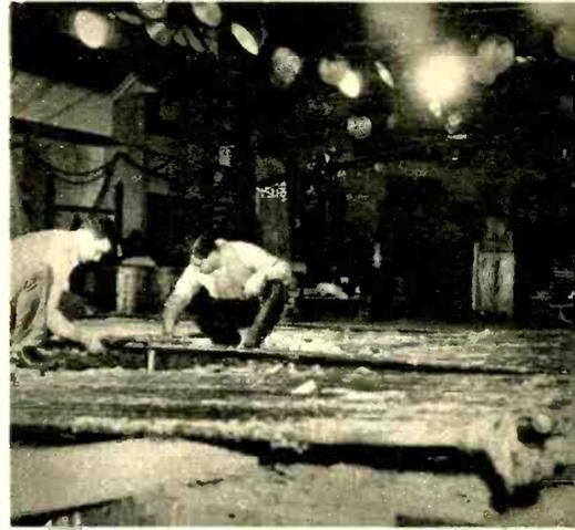
1. Warm TV lights—cold ice. The combination brought problems. Workmen had to cut pipes in half before installing them.
