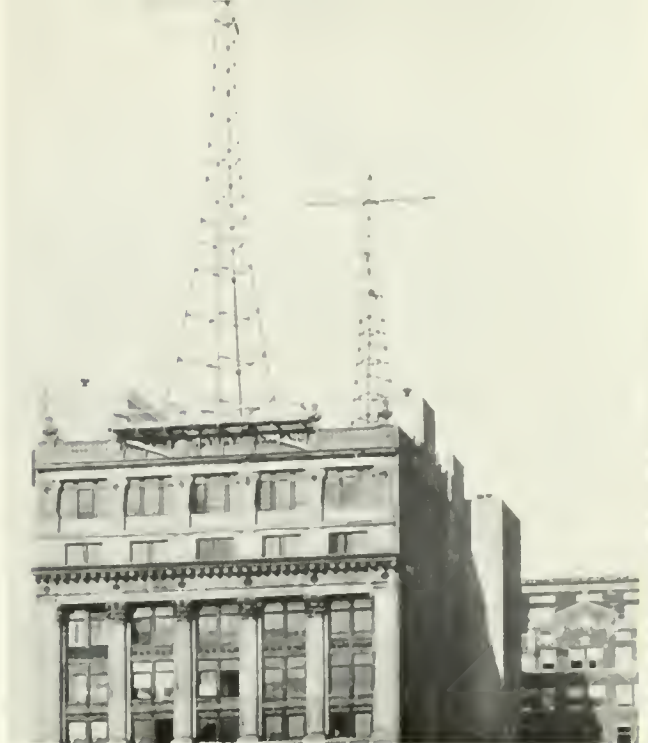
Dual antennas for stations WJZ-WJY were erected on the roof of Aelion Hall in New York City.
