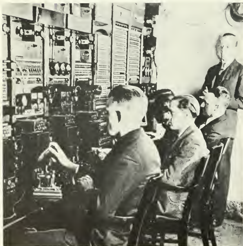
NBC's first radio program was put on the air November 15, 1926, from this main control room in the A. T. & T. Building, New York City. O. B. Hanson, then NBC Chief Engineer, now Vice President and Chief Engineer, stands in the rear.
