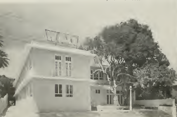
BELOW: MODERN, AIR CONDITIONED HOME OF STATION WJAC IN SAN JUAN, PUERTO RICO.
