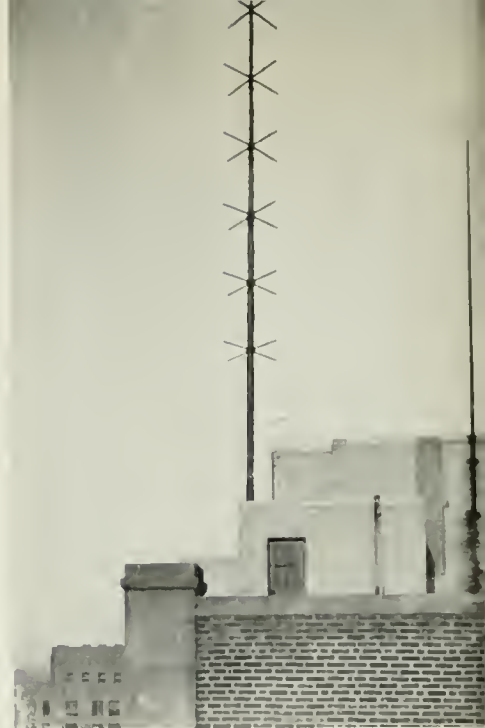
“TURNSTILE” ANTENNA USED WITH THE FM TRANSMITTER OF STATION WCAU, IN PHILADELPHIA.
