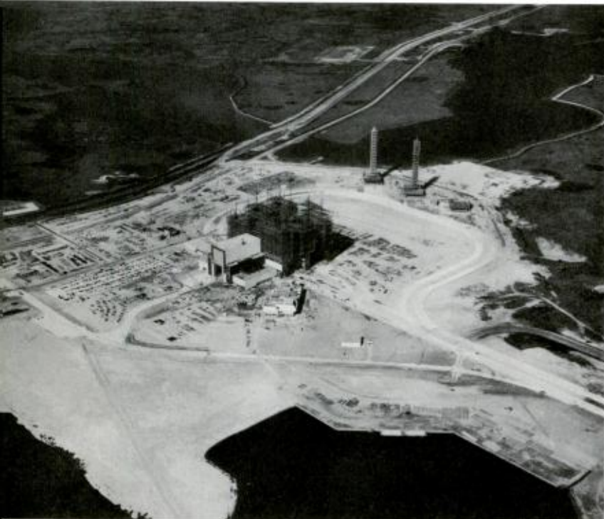
Aerial view of NASA's Spaceport on Merritt Island, Fla. Since photo was taken, steel work has been completed on the third of the Mobile Launchers, shown at center right.
