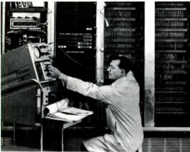
testing of the line buffer/scanner . . .
