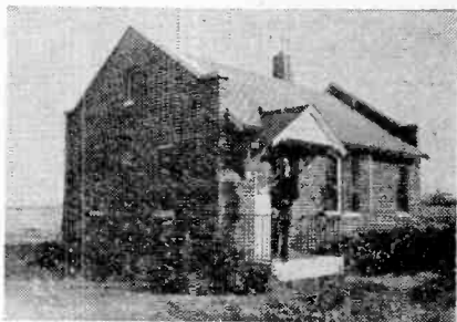
The transmitter building of WTRC, Elkhart, Ind. DXer Roger Malt, who submitted the picture, is standing in the doorway.
