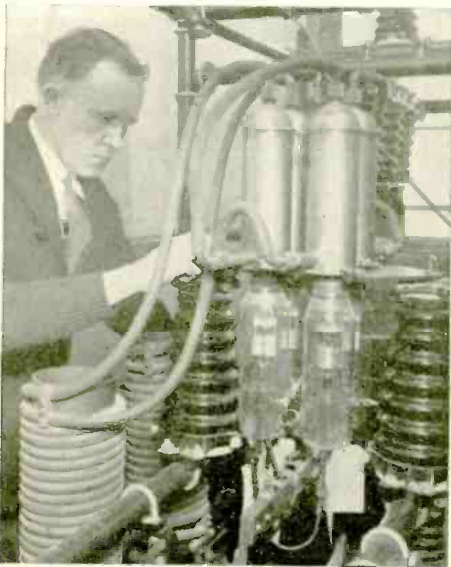
Four of the 64 ten-kilowatt tubes that are used in the station. The water-cooling jackets and tubing are here shown.
