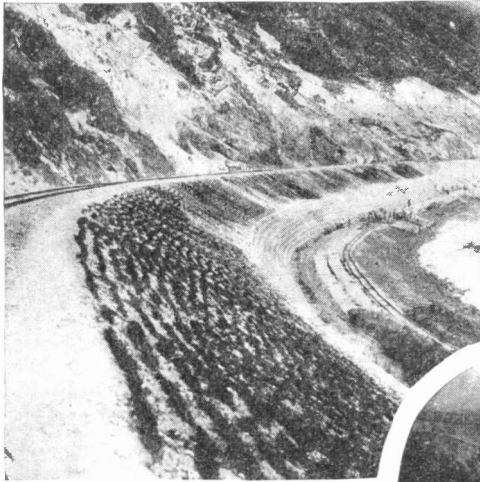
Native Grass Planted on an Embankment to Prevent Erosion
