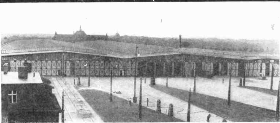
Largest car barns in the world; built at Lichtenberg by the Berlin Street Railway Co. The barns are approximately 2,850 feet long by 360 feet wide and contain track space for 500 cars at one time.
