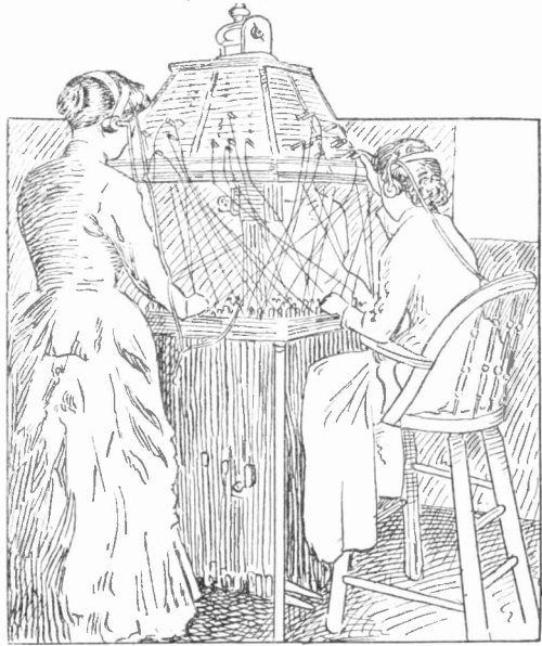
A Telephone Switchboard used 31 Years Ago—Drawn from a Photograph
