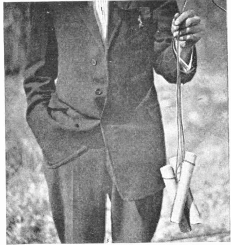
DYNAMITE CARTRIDGES READY FOR DITCH DIGGING
