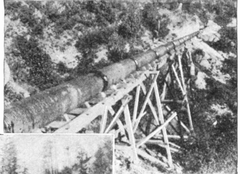
A SECTION OF THE WOODEN PIPE LINE
