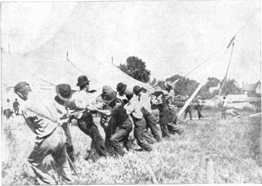
RAISING THE CENTER POLE WHICH CARRIES THE ELECTRIC CABLES
