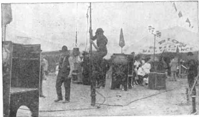
BURYING ELECTRIC CABLE ON THE CIRCUS GROUNDS
