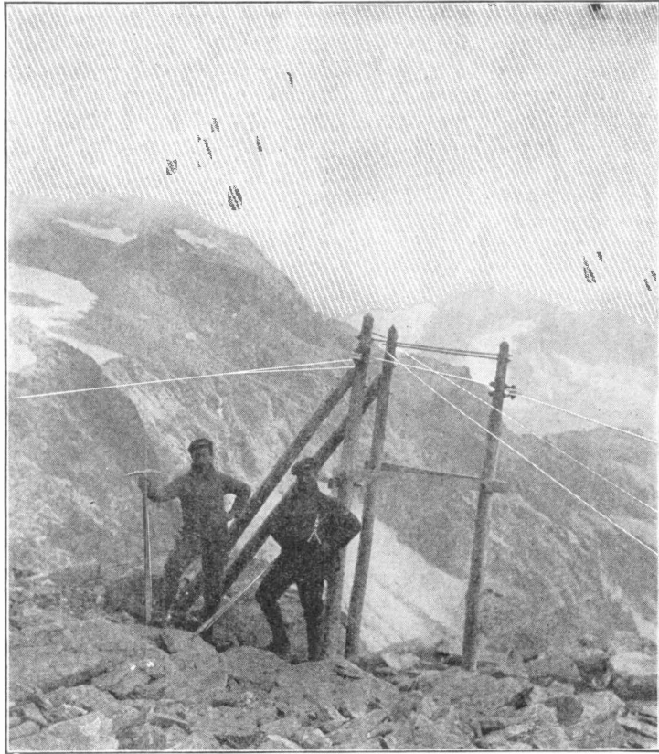
HEAD END OF WIRE SPAN MORE THAN 1100 YARDS IN LENGTH
