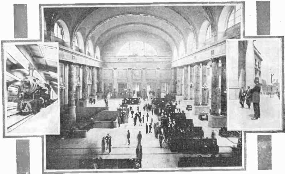
MAIN WAITING ROOM OF THE NORTHWESTERN RAILWAY TERMINAL
