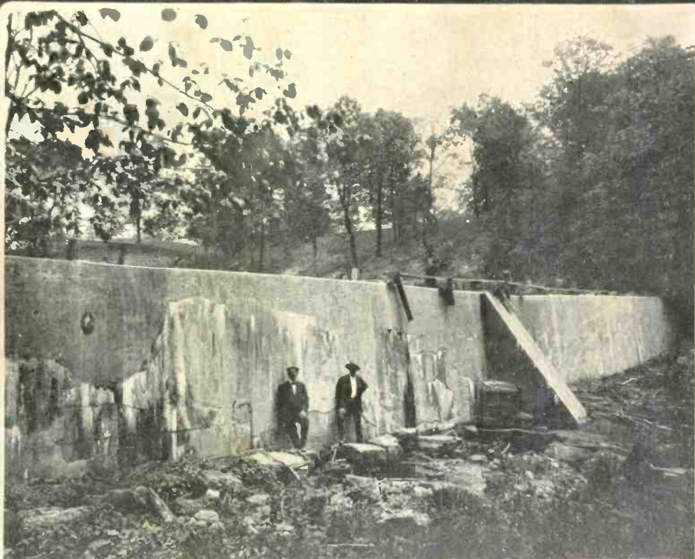
CONCRETE POWER DAM ON THE ELECTRIC FARM
