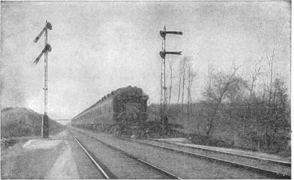
FIG. 18. THIS TRAIN HAS PROTECTED ITSELF—RIGHT-HAND SEMAPHORE INDICATES "STOP" TO FOLLOWING TRAINS
