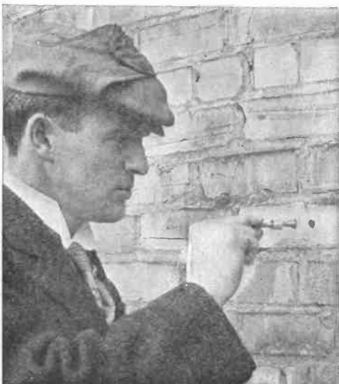
THE BOLTS ARE INSERTED HEAD FIRST
