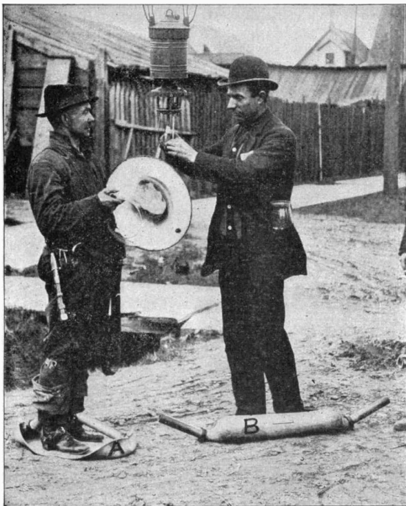
USING "SHIELDS" IN TRIMMING ARC LAMP
