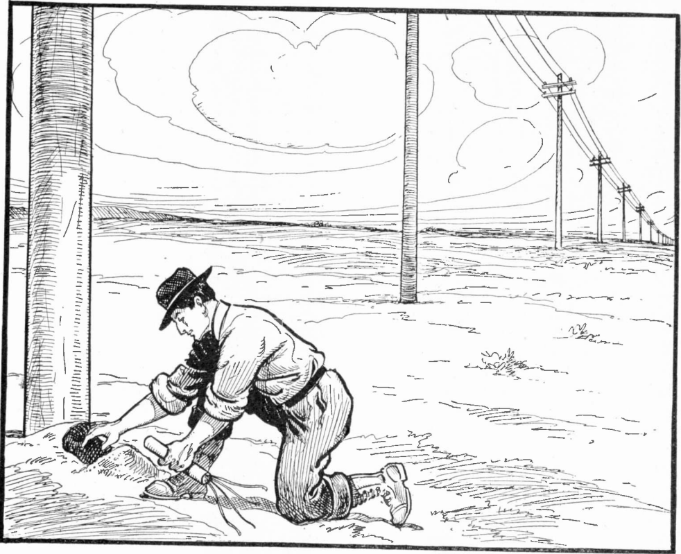
HE UNEARTHED SOME IRON-CLAD COILS.
