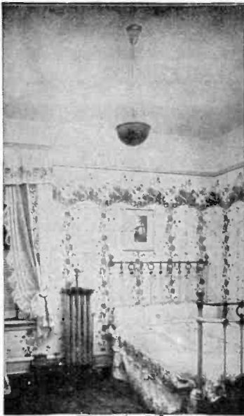
Room 12x14 feet, beautifully illuminated with a one-unit fixture containing one 60 watt Tungsten lamp—consuming current about equal to one 16 c. p. carbon filament lamp.
