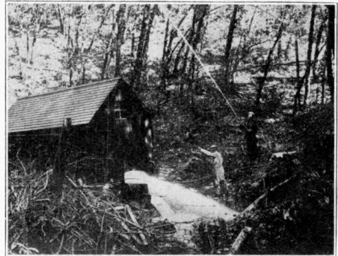
POWER PLANT IN OPERATION.
