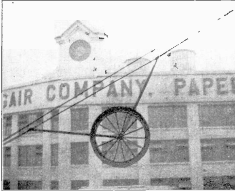
FIG. 2. TRAVELING SHEAVE.
