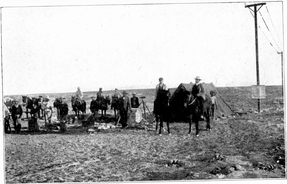
ERECTING A TRANSMISSION LINE THROUGH THE DESERT.
