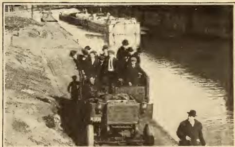
Electric Truck Towing Three Canal Boats, Representing a Load of 731 Tons
