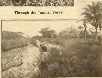
A Cutting in Mombasa, the Start of the Railway
