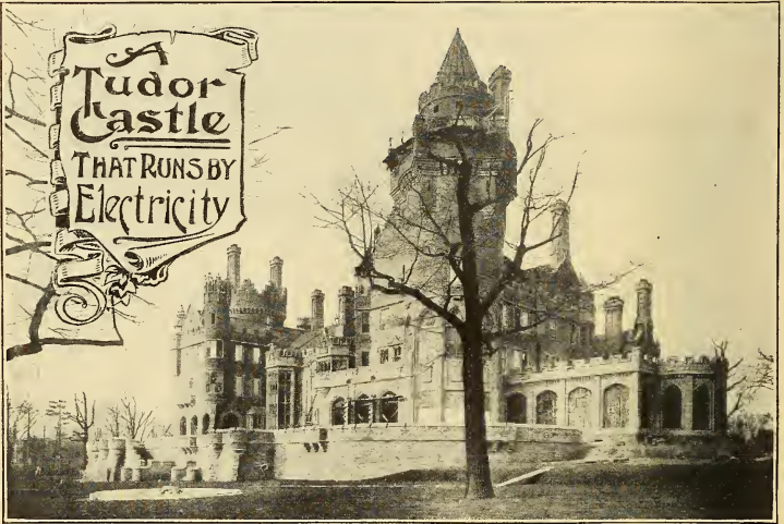
The Castle of Sir Henry Pellatt, in Toronto, Built at a Cost of $1,500,000
