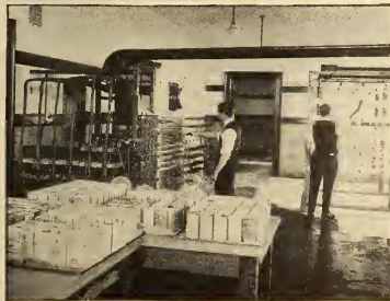
The Lamp Room where 5000 Lamps a Year are Burned Out in Life Tests
