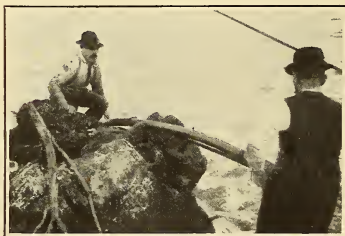
Laying a Submarine Cable
