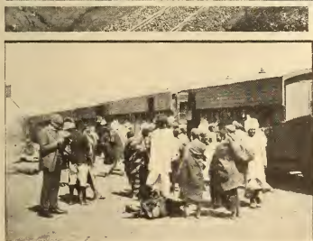
A Railway Station on the Uganda Railway
