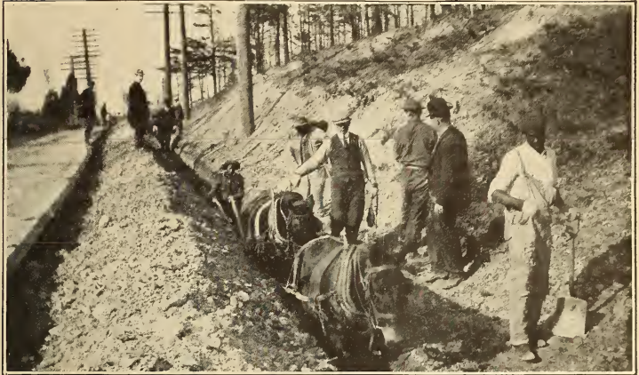
Plowing a Trench between Baltimore and Washington
