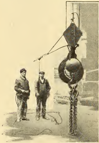
Fig. 2. Signal Man Operating Hoist
