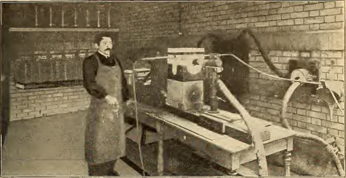
ELECTRIC FURNACE USED BY PROFESSOR MOISSAN IN MAKING DIAMONDS
