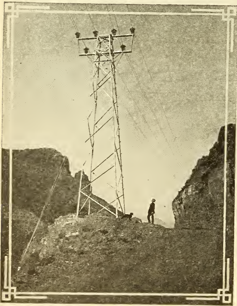
ALONG THE TRANSMISSION LINE, JUST BELOW THE ROOSEVELT DAM
