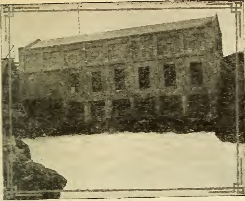
MINIDOKA POWER PLANT IN IDAHO
