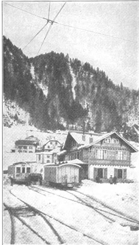
STATION AT LES AVANTS
