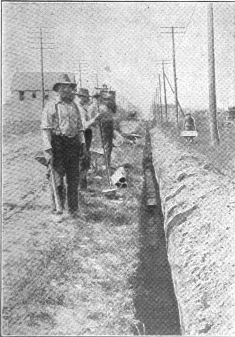
UNDERGROUND WORK WHICH MADE NECESSARY THE PUPIN COIL
