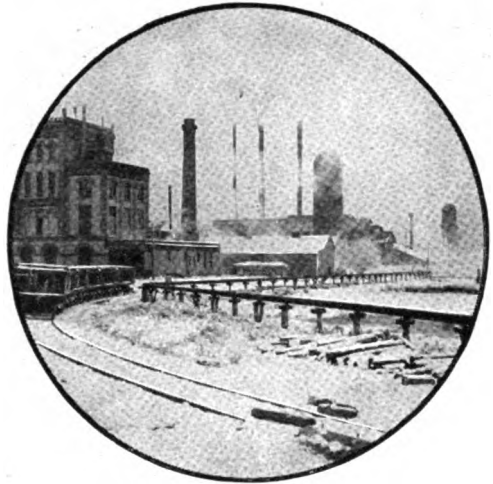
PART OF THE 2100-FOOT PIPE LINE
