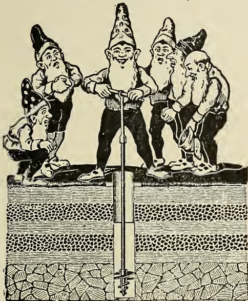
LINE CONSTRUCTION IN ELFLAND
