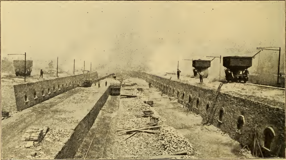
FIG. 1. ELECTRIC CHARGING OF COKE OVENS.
