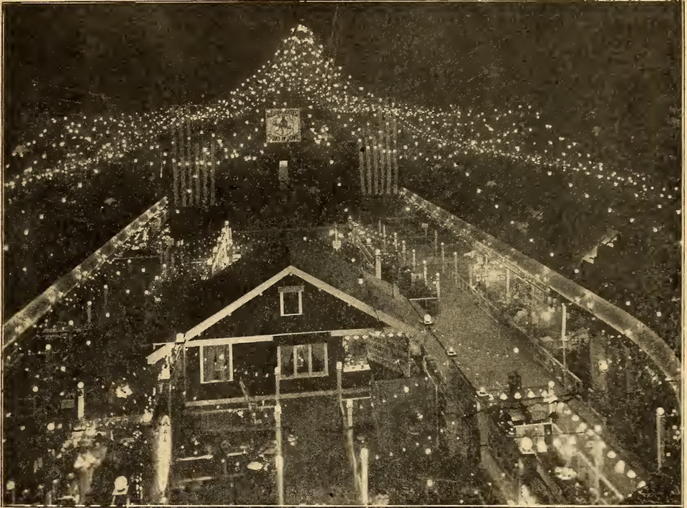
OMAHA ELECTRICAL SHOW.
