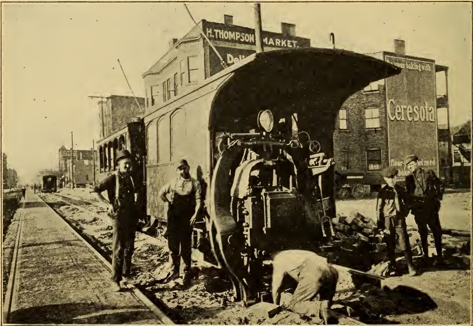
ELECTRIC RAIL WELDING CAR.
