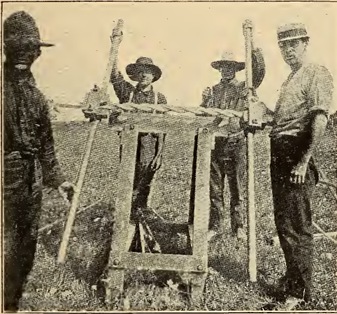
FIG. 5. SPLICING THE ALUMINUM CABLE.
