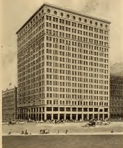
FIG. 1. MODERN SKYSCRAPER WHERE ELECTRICITY IS A WONDER WORKER.
