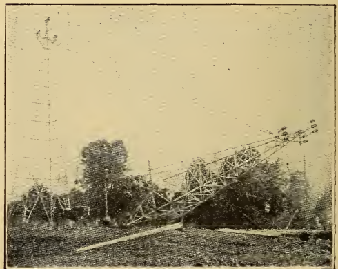
FIG. 4. RAISING A TOWER.
