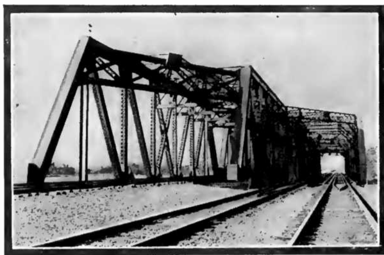
A Graphic Illustration of the Changes Wrought During a Period of Twenty-Five Years In the Design of Bridges.
