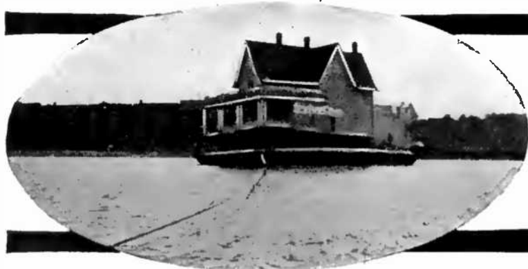
Moving a House by Means of a Large Scow Results in a Time and Monetary Saving if the Dwelling Is Located Near a Waterfront.
