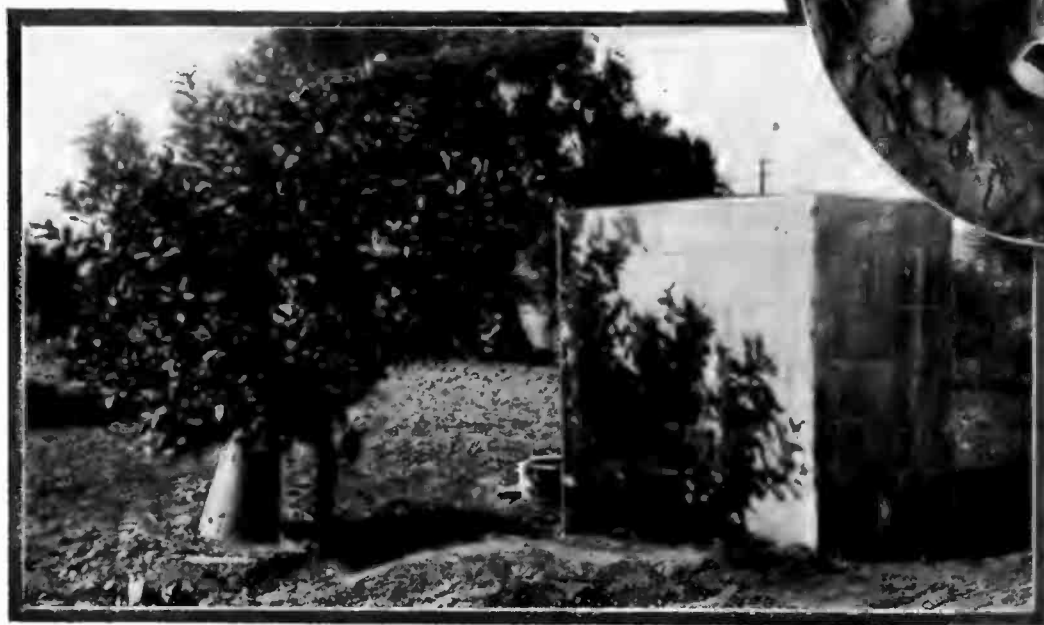
At the Left: The Pressure Box of the New Concrete Irrigation System. Above: One of the Concrete Stations with Connecting Pipes.
