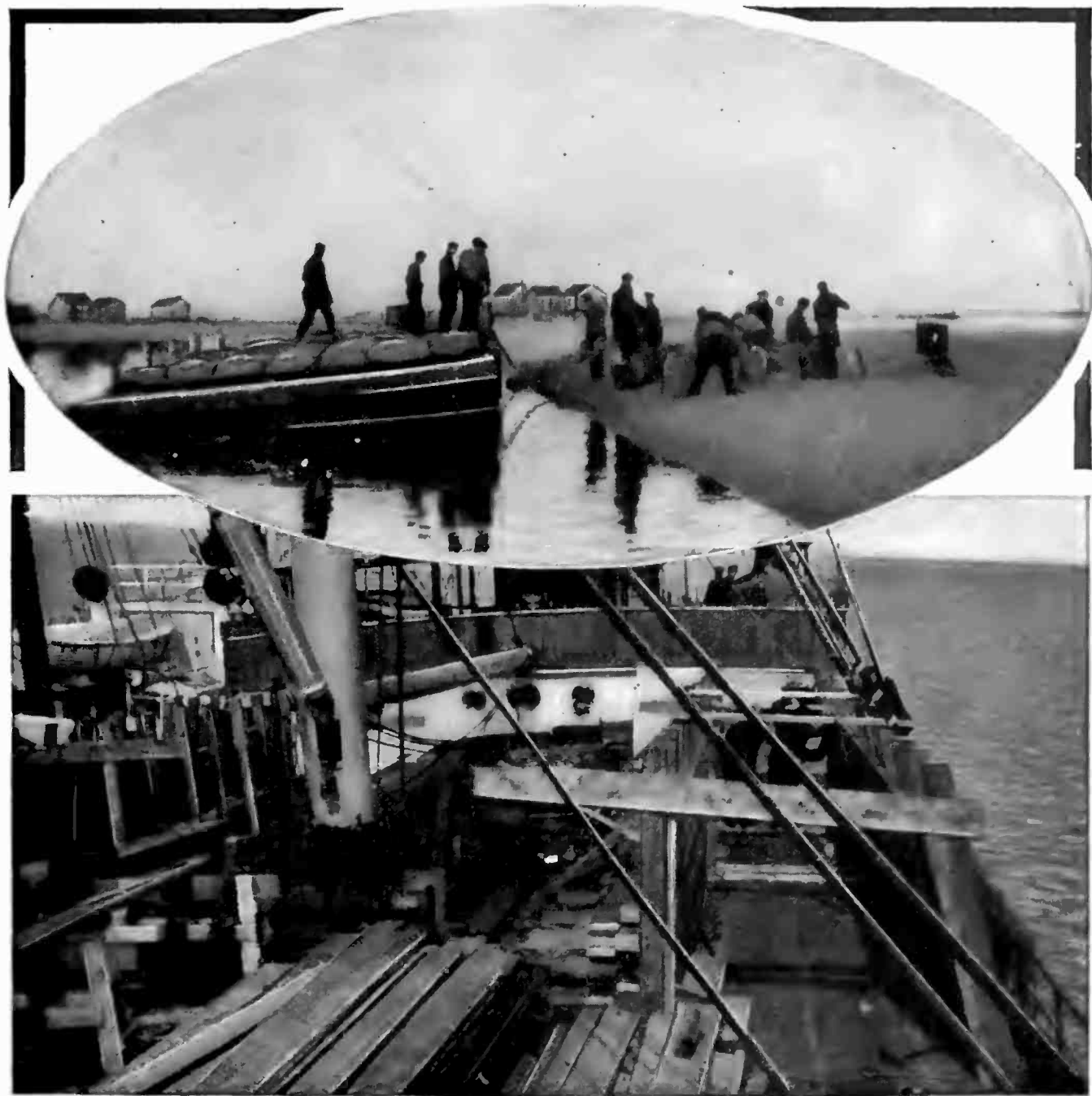
In the Oval: Loading the Sand Bag Ballast On a Barge In Order to Transport It to the Steamer. Below: How the Righting Tanks Were Built Quickly Upon the Deck of the Steamer "Berlin."
