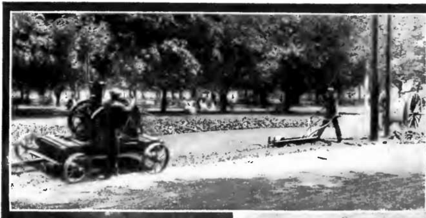
Two Views of a Newly Devised Plow that Lays Cable Underground. In One View May be Seen the Complete Equipment, and in the Other the Plow Alone.
