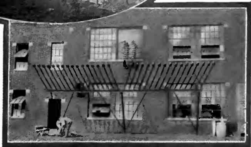
At the Right: Foot of the Aerial, Where the Lead-in Wires Are Brought Into the Transmitting Station. There Are Thirty-two Wires in All.
