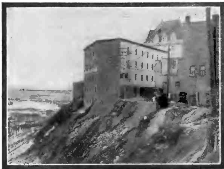
Landslides have Carried Away Most of the Main Street of Edmonton, Canada, and are Now Threatening Buildings.
