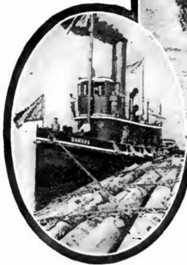
A Huge Log Raft Being Towed from Oregon to Southern California. This Method of Transportation Effects a Great Saving in Cost as Compared to Rail Shipment.
