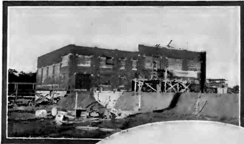
At the Left: Power House at New Brunswick in Course of Construction. In the Oval: Auxiliary Operating Building at New Brunswick.
