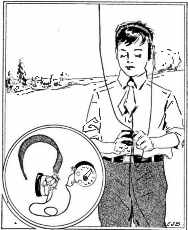
A Pocket Wireless Set Containing a Tuning Coil and Crystal Detector.
