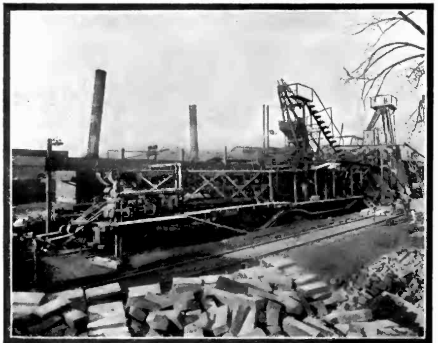
By means of Conveyor Belts on this Long Car, the Finished Blocks are Carried Through 150 Feet of Cold Water.
