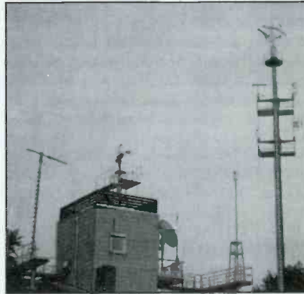
Chris Halinar came across this interesting U.S. communications site while traveling through Germany.
