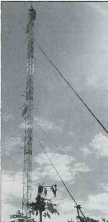
This tower belongs to FR3, Noumea, New Caledonia.
