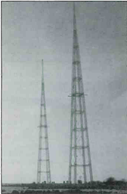
The Swedish mediumwave station at Solvesborg on 1179 kHz. The transmitter runs 600 kW and these towers can effectively pump that up to 2000 kW east-west directional. At night, the signal covers an area populated by 165 million people.
