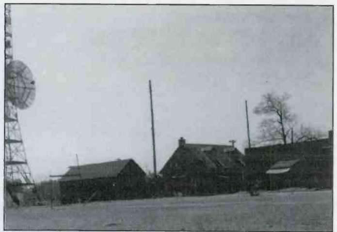
Another view of the abandoned Riverhead RCA receiving facility. Note the large (west-facing) microwave dish at the left.
