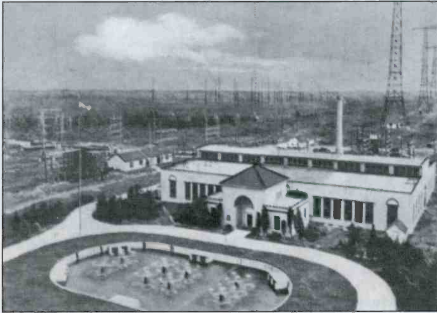
Radio Central's transmitter building and cooling pool, with antenna farm, as they looked from the air in the late 1930s.
