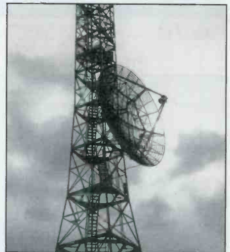
A better look at the abandoned RCA microwave tower and dish at Riverhead.
