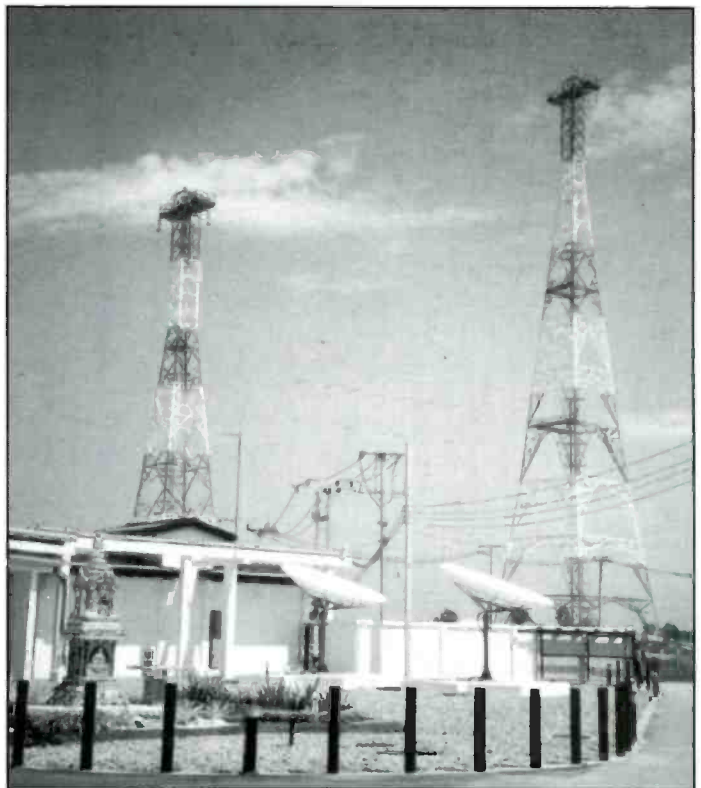
↓ Masts at the BBC Asia Relay Station, Nakhon Sawan, Thailand.
