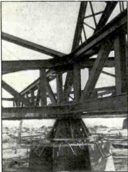
This photo shows the PCJ revolving beam antenna system's iron pivot partly sunk into a concrete foundation. The whole system of undercarriers rotated around this pivot, united by a steel bridge.
