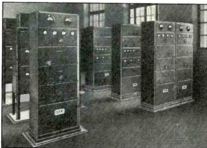
← A view of the complex speech processing and amplifier panels that could scramble voice transmissions for privacy.
