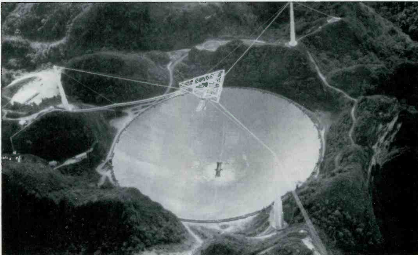
The National Science Foundation's 1000-foot diameter radio telescope near Arecibo, Puerto Rico listens to tiny segments of the universe for signals from advanced civilizations.
