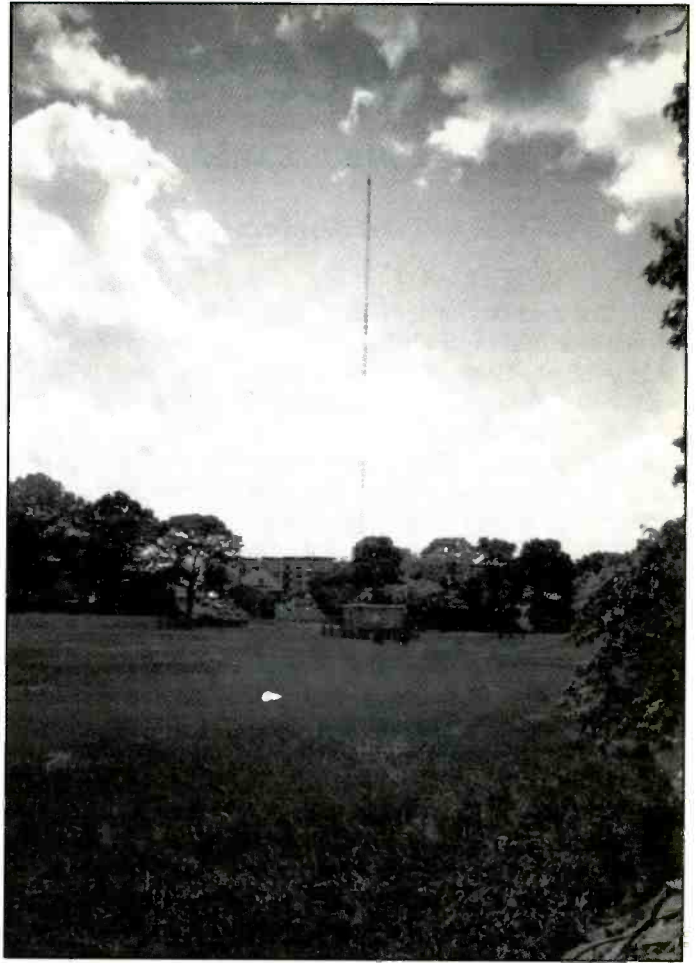
Quincy, Mass. station WJDA-AM has its transmitter and antenna located in a salt marsh, which makes for good ground conductivity, but poor accessibility during high tide. (Courtesy an anonymous reader)
