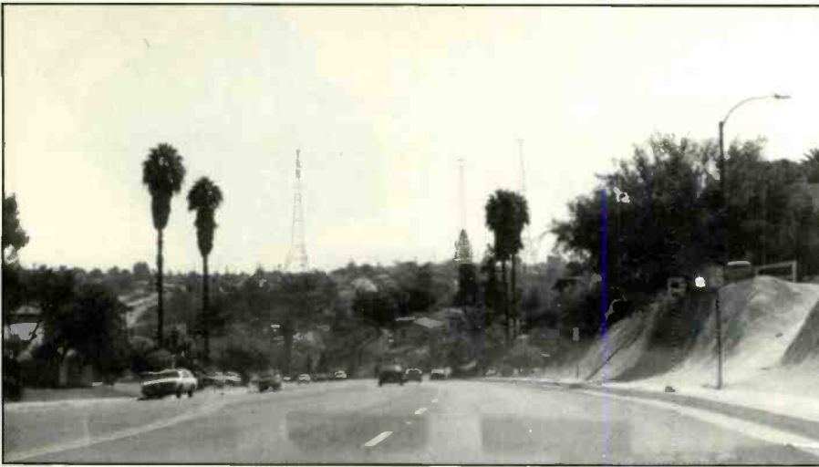
This long shot of the San Diego installation shows all three towers.
