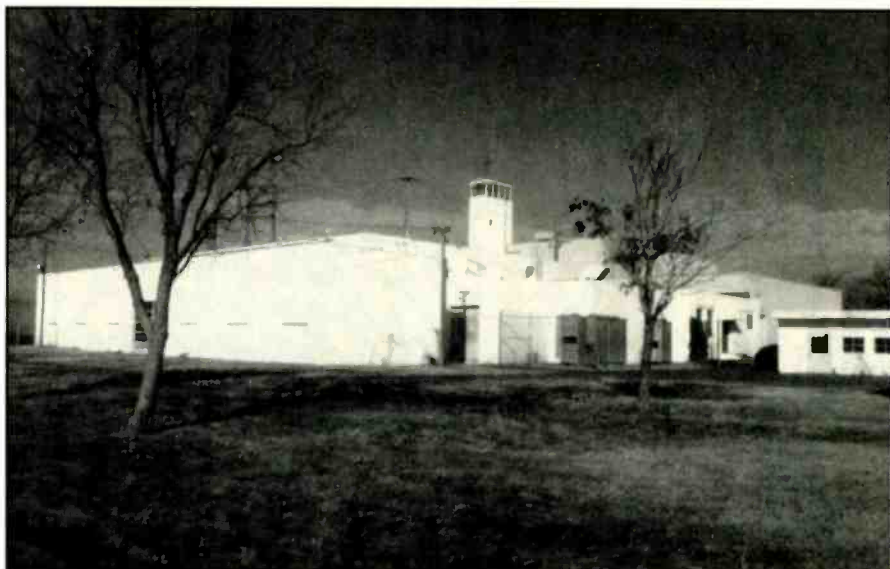
Rear side view of main building of the former VOA station. The tower on the building was apparently a security feature. Note the high voltage enclosures behind small tree, right of center.
