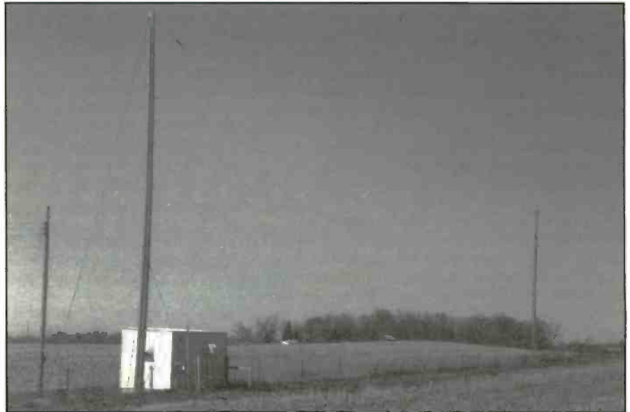
Ralph Craig of Ohio provided these photos of beacon antennas. This one is CCJ, 341 kHz, Springfield, Ohio (just east of the airport). It is an inverted L, 200 feet long.
