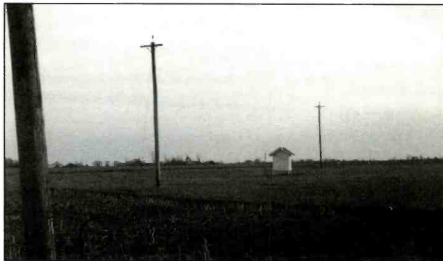
Oxford, Ohio, (Miami University) is the location of Beacon OXD, 282 kHz. The T antenna is about 200 feet long. The small white building houses the transmitter. Typical installation of low-cost "h," state owned.
