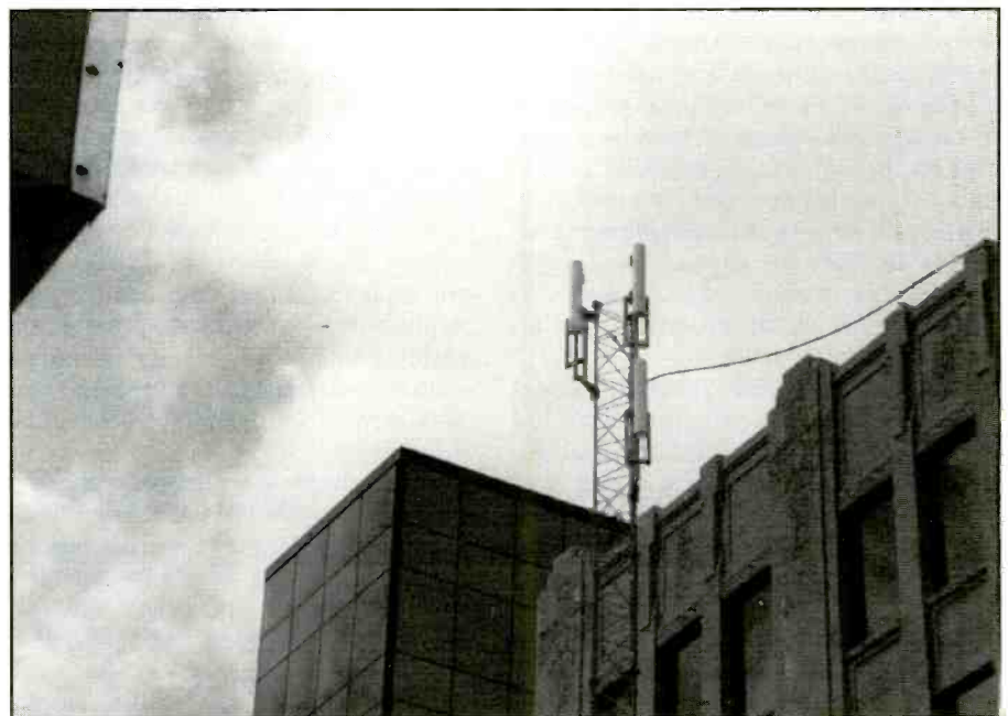
These are the antennas at the top of the tower on the FEMA repeater trailer in Oklahoma City. (Photo by Dick Sharp)
