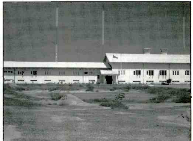
The Puttalam transmitting site in Sri Lanka.
