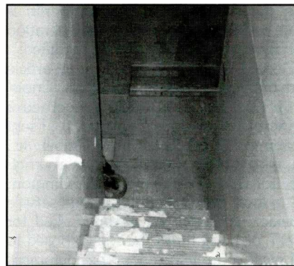
Stairway from ground level offices and checkpoint down to underground bay.
